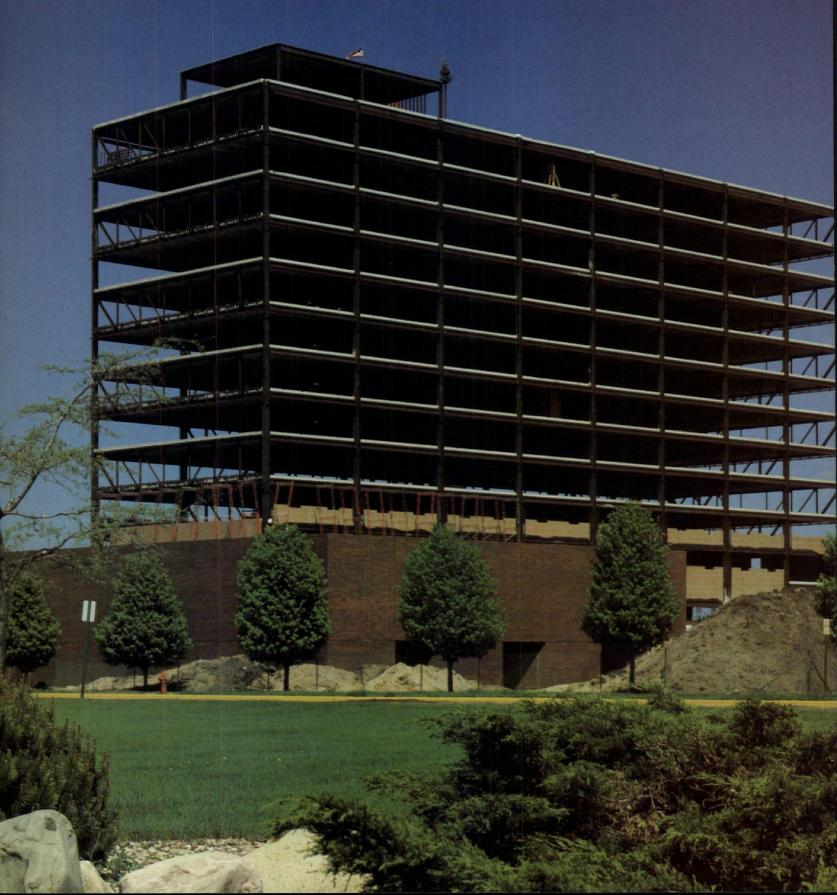
Many high-rise apartments and hoteltype structures have been built with the Staggered Truss steel framing system. It allows efficient and economical use of structural steel, with great flexibility and erection speed.
