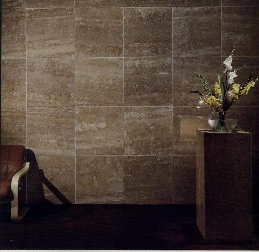
WALL - GL MARBLE - ST. PETER TRAVERTINE POLISHED 2'x 2'x 1/4" THICK INSTALLED WITH THIN-SET ADHESIVE OVER GYPSUM WALLBOARD
