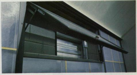
Detail of the Trombe wall from the outside. Manually operated windows can be opened if necessary. This picture shows the class room ventilators which are opened or closed automatically by thermostats, and the black painted concrete masonry Trombe wall.
