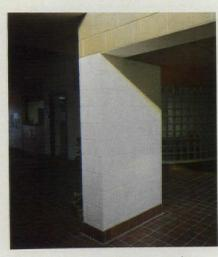
Loadbearing concrete masonry is employed throughout the structure.
