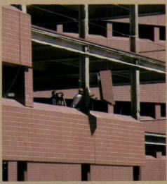
PRUDENTIAL INSURANCE CO., Philadelphia, PA. Prefabricated 20' x 7'4" panels of 4" x 8" Gail Unglazed Brickplate being installed at jobsite by Duggan & Marcon. Arch.: Ballinger Co., Phila. Gen. Contr.: Daniel J. Keating Co., Villanova, PA.
