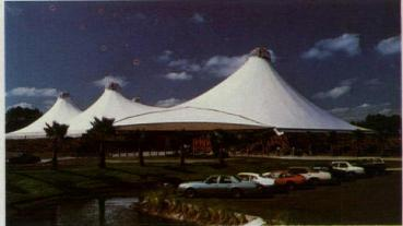
"Florida Festival" in Orlando, Fla., has the highest light transmission (18%) yet developed for a roofing fabric. The permanent structure is a free-form tension canopy made of Fiberglas" fabric coated with DuPont TEFLON fluorocarbon resin. The 60,000 sq. ft. complex is designed to provide recreation, entertainment and a bustling marketplace attraction for the millions who visit Sea World Park each year.
