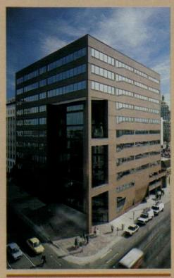
SPECTRUM BUILDING, Denver, CO. Gail Unglazed Brickplate, 4"x 8" on prefabricated panels for exterior walls. Architect: McOG Associates, Denver. Gen'l Contr: Turner Const. Tile Contr.: Ace Tile, Denver.
