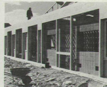
Left: A bank of photovoltaic cells, mounted in an adjustable collector, powers insulating curtains and air-circulating fans. Below: Trombe wall under construction. Bottom center: Plastic cylinders filled with water store heat during the day. Bottom right: Light reflected in roof monitor bounces onto mirror strips and masonry wall.
