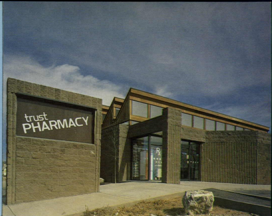
The entrance to the pharmacy, showing the series of clerestory windows providing both lighting and solar heating. The structure is faced with split ribbed concrete masonry units, accented with split block.
