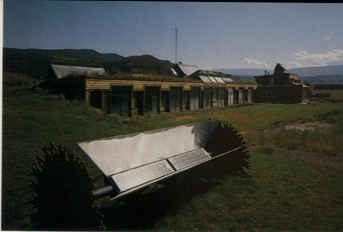
Left: A bank of photovoltaic cells, mounted in an adjustable collector, powers insulating curtains and air-circulating fans. Below: Trombe wall under construction. Bottom center: Plastic cylinders filled with water store heat during the day. Bottom right: Light reflected in roof monitor bounces onto mirror strips and masonry wall.
