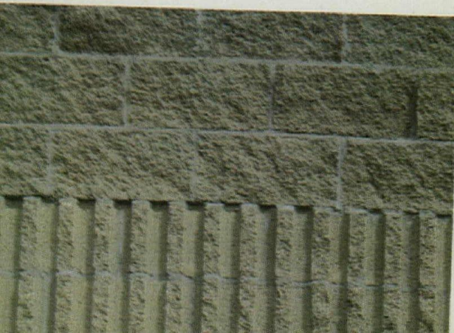
Wall detail showing how the concrete split ribbed and split block units are employed in the design.
