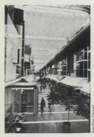
Students' Union Housing, Edmonton, Alberta, 1972: Architects: A.J. Diamond & Barton Myers; R.L. Wilkin, associated architect. A glazed internal street, with adjustable shading and venting controls; maintained at lower temperatures, the space is essentially heated by gains from surrounding spaces.
