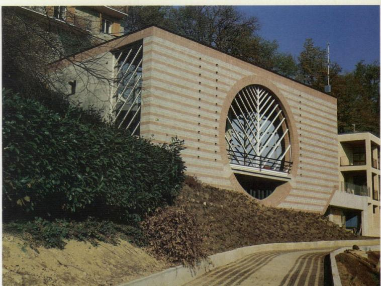
In many ways the house in Massagno (1981, above) is similar to the one in Viganello. There is a long approach path, here paved in concrete block with grass growing through. There is a piano nobile arrangement, and rooms are distributed around a central double-height greenhouse with sliding glass panels facing the best view. As at Viganello, there are air and light shafts-two, both on the west side of the building. But unlike Viganello, entry is not under the greenhouse but on the north side.
