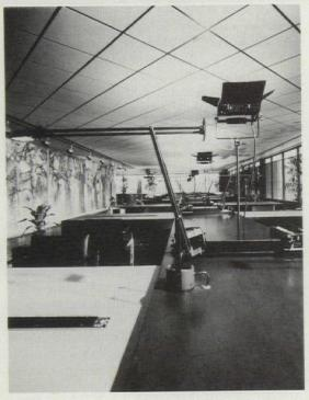
Project: Ridgway Ltd. offices, Newport Beach, Ca. Architects: Ridgway Ltd. Program: approximately 6000 sq ft of office space, with reception, conference, and work areas. Mechanical systems: air supply and return through continuous slot at joint between gypsum board and ceiling tile. Major materials: gypsum
