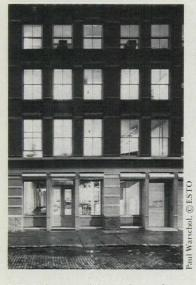
View of restored front shows three Knoll floors plus one of three stories of apartments. New doors and insulating windows reproduce look of originals; groundfloor roller doors provide sleek counterpoint.
