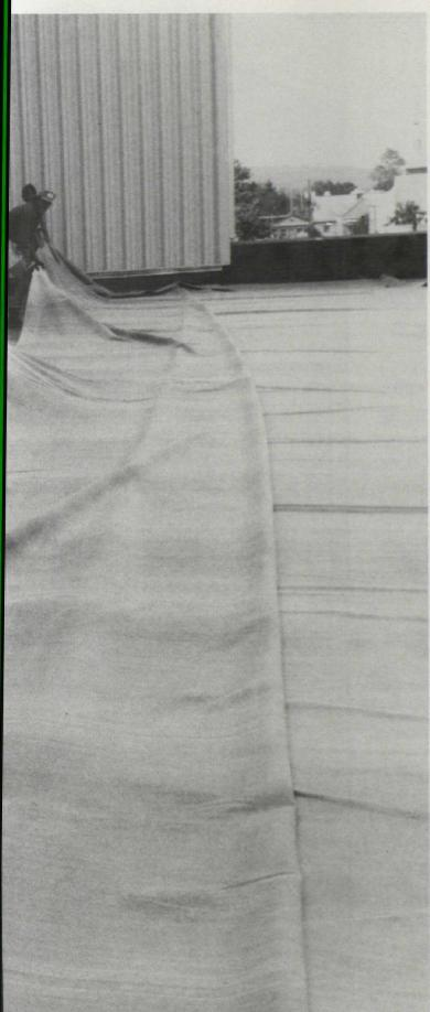
An experienced roofing contractor will usually install a quality single-ply rubber roof in about half the time it takes to cover the same area with built-up roofing. The table below shows the average number of squares laid per-man, per-day as reported by single-ply and BUR roofing systems suppliers and contractors:
