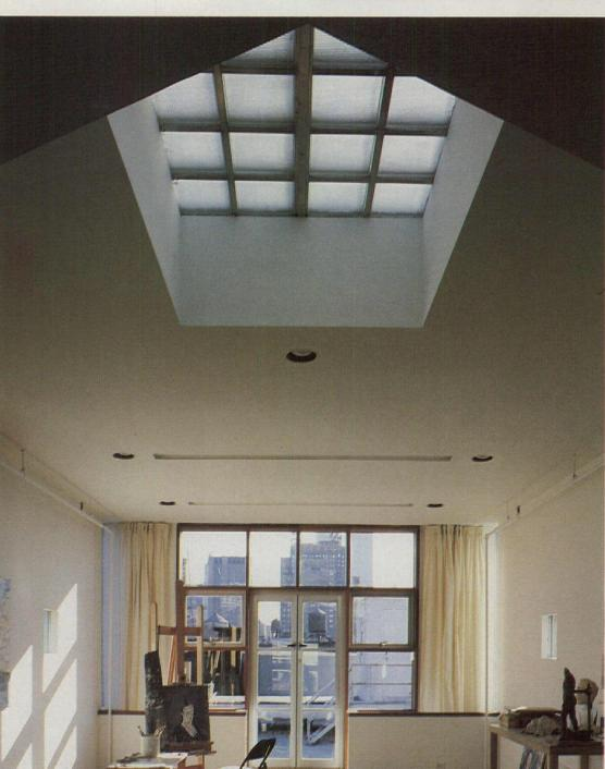
Together with the skylight overhead, triangular panels of glass seem to cut the "apse" (above) free of the surrounding volume. Access to the roof is from the south end of the studio, where light bounces down below through slots below the railings.
