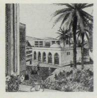
The King Abdul Aziz University in Mecca, Saudi Arabia, by SOM employs several arid climate design strategies: massive walls for thermal lag, wooden screens for shading, vegetation for humidification, louvered blinds for ventilation, light surfaces for reflectance, and courtyards for trapping night air.
