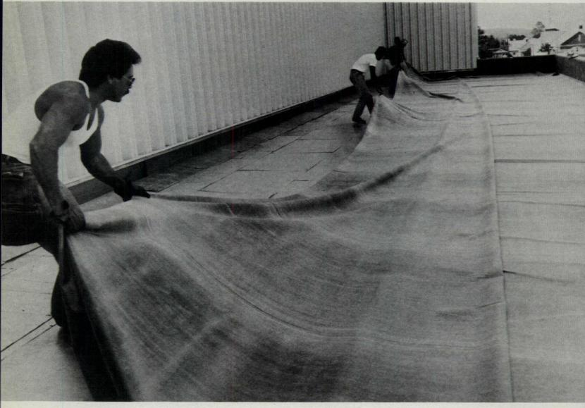
An experienced roofing contractor will usually install a quality single-ply rubber roof in about half the time it takes to cover the same area with built-up roofing. The table below shows the average number of squares laid per-man, per-day as reported by single-ply and BUR roofing systems suppliers and contractors:
