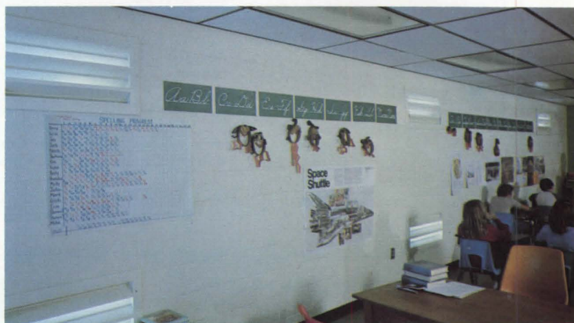
The classroom side of the Trombe wall, showing vents, through which solar heated air enters the room.
