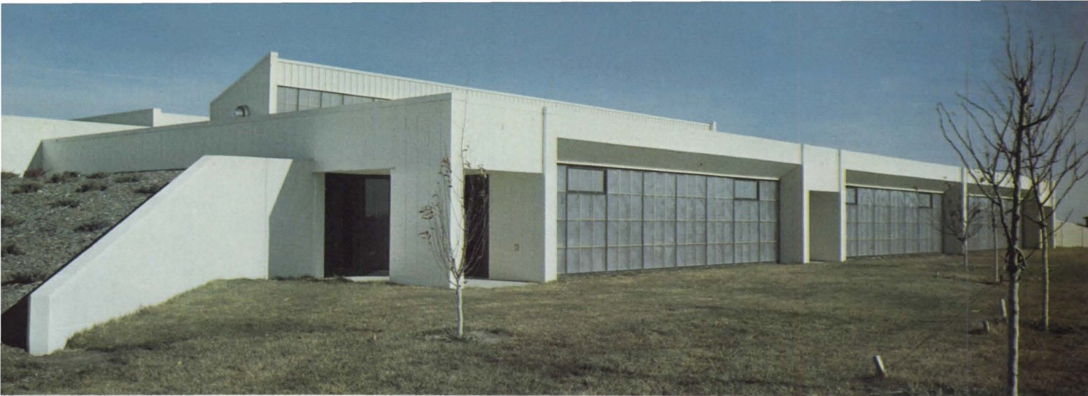
View of the school from the south showing the 160' Trombe wall.
