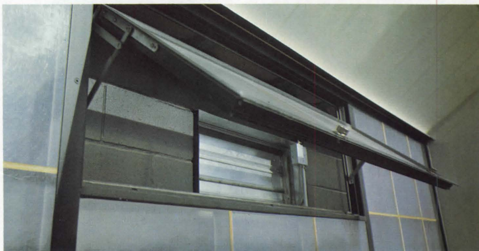
Detail of the Trombe wall from the outside. Manually operated windows can be opened if necessary. This picture shows the class room ventilators which are opened or closed automatically by thermostats, and the black painted concrete masonry Trombe wall.
