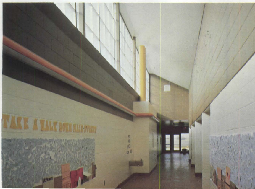
A view along one of the axial corridors showing the clerestory windows and the solid concrete masonry heat storage wall.
