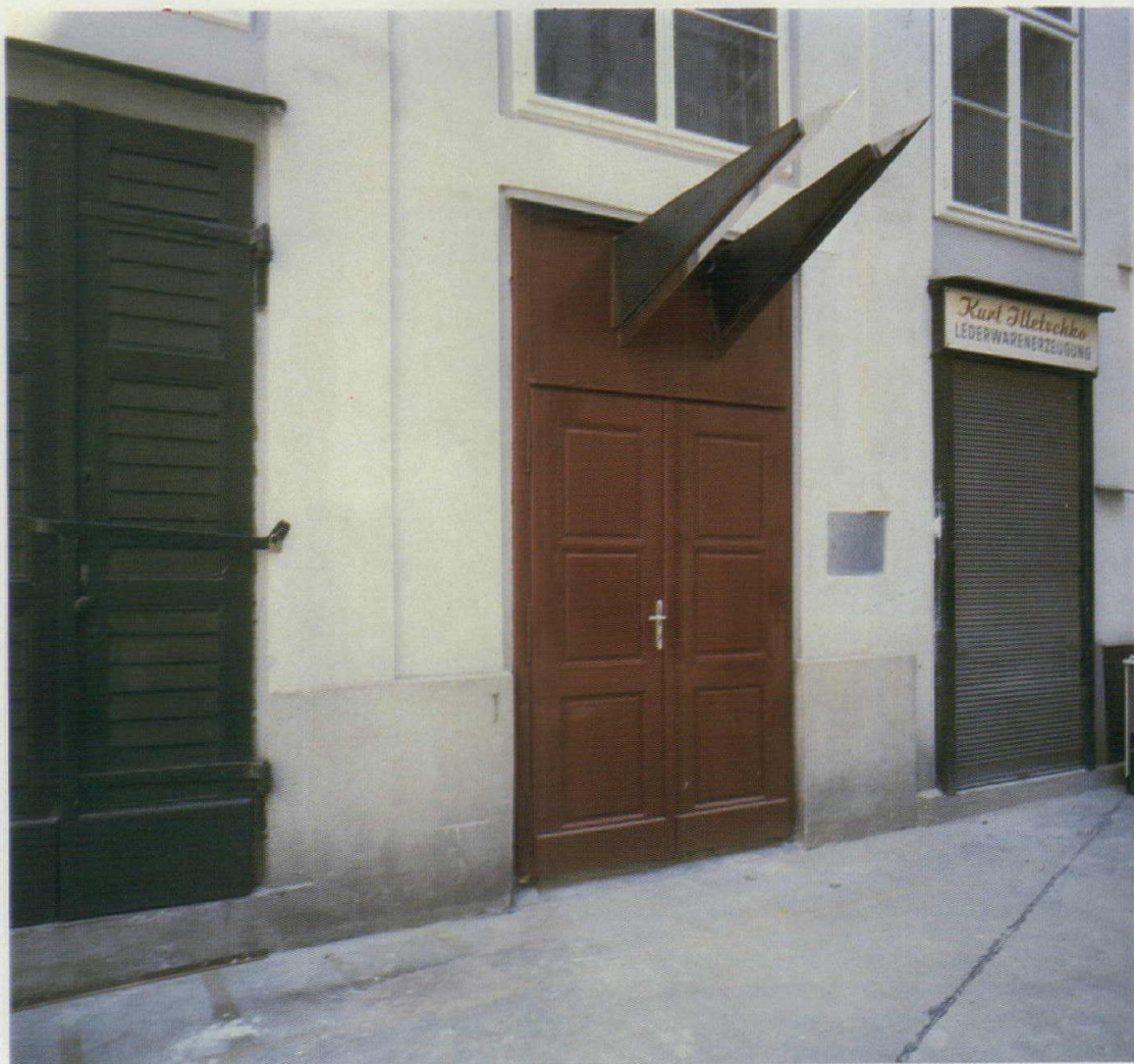
Project: Der Rote Engel Bar, Vienna. Architects: Coop Himmelblau, Vienna (Wolfgang Prix, Helmut Swiczinsky, partners). Program: a wine bar and performance hall, seating 120, in a 1300-square-foot space on the ground floor of an 1835 landmark structure. Major materials: stucco vault, corrugated tin doors and wall cladding, concrete ledges, red pine shelves and countertop, asphalt floor. Glass block, plaster, tin, and stainless steel "angel." Photography: Gerald Zugmann.
