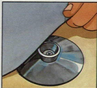
1 Roll membrane over knobbed base plate.
