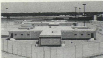
Modular correctional facility, Leesburg, N.J.
