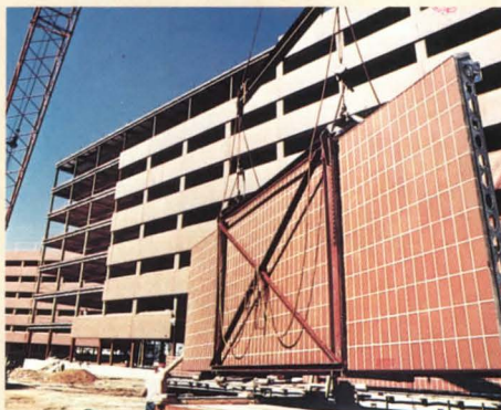
Panels being installed at the Prudential Insurance Company, Philadelphia, Pa. by Duggan & Marcon using Gail Brickplate and H.B. Fuller Latex Modified Mortar. Arch: Ballinger Co., Phila. Gen. Contr.: Daniel J. Keating Co., Villanova, Pa.
