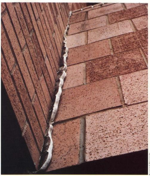
The failure of a wall joint almost always indicates either poor detailing or poor construction (See P/A Practice, p. 57). Many problems occur with joints made too narrow to accept a sealant or to accommodate the movement of adjacent materials, leading to the squeezing of the sealant from the joint (above). Remedial action might include widening the joint to make more room for the sealant or applying a "band-aid" joint.
