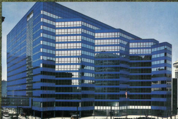
2500/3000 IB Wall. Minimum metal requirements allow a flush grid appearance with superior windloading and interior erection and glazing.
