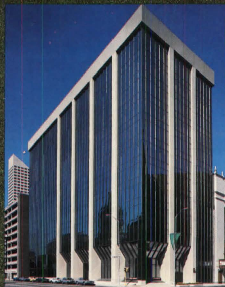
Stickwall 8000. Exterior projected vertical mullions for vertical design emphasis with interior pressure glazing tested to meet or exceed ASTM curtainwall standards for air, water and structural performance.
