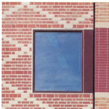
A window in east end wall is linked by a painted metal strip to a band of dark brick on abutting long wall.
