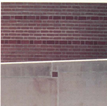
On handicapped ramp parapet (bottom left in drawing) a tile inset reconciles levels of limestone slabs.
