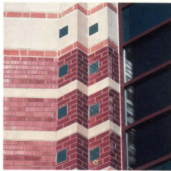
A south entrance (top in drawing) is framed by facets of glazed and unglazed brick, limestone, and tile.
