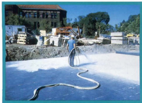
A two-part bentonite is then sprayed over the rubberized asphalt.
