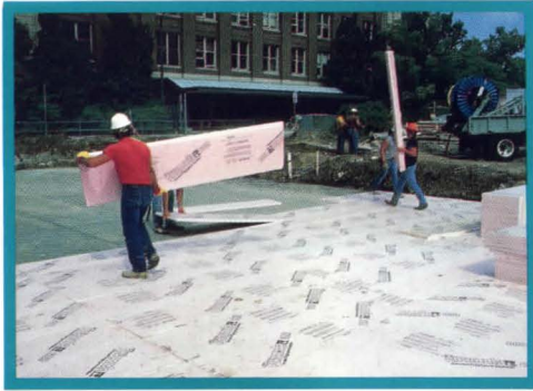
A high density extruded polystyrene insulation goes over the EPDM.
