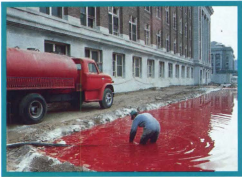
The red food coloring highlights any leaks during the 48-hour test.
