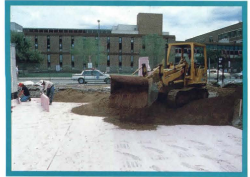
Free-draining backfill is then carefully placed over the insulation.
