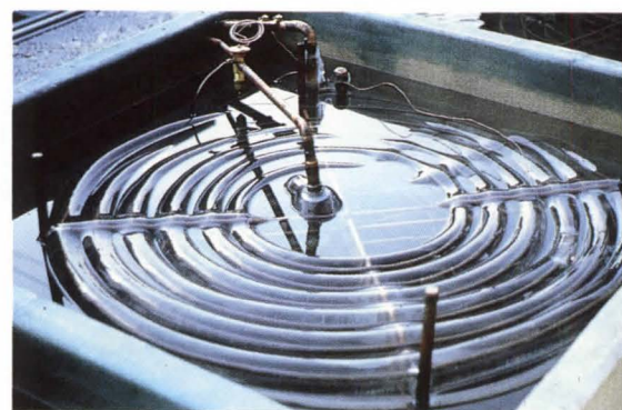
Thermal storage coils used at Florida Power & Light, Pompano Beach, Fla.
