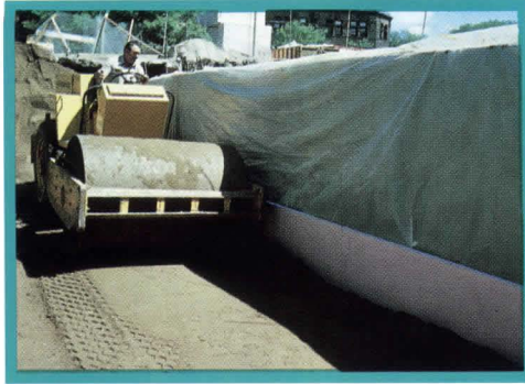
Free-draining backfill is laid against extruded polystyrene insulation.
