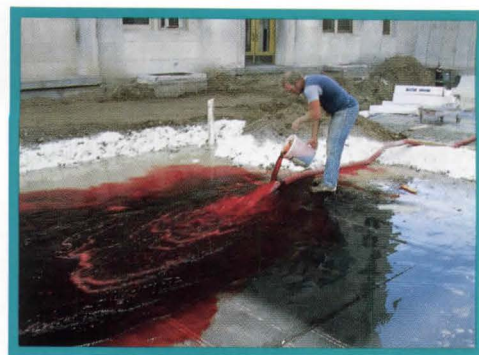
The contractor adds red food coloring to water during the flood test.
