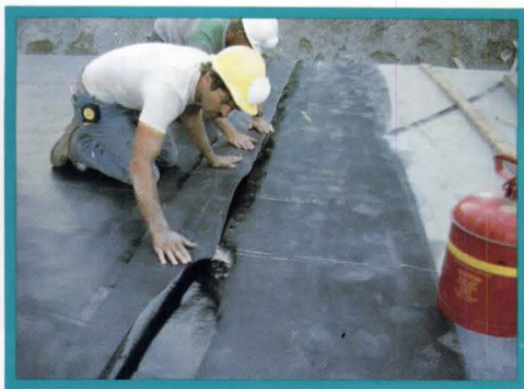
Workers join the top layer of EPDM sheets with contact adhesive.
