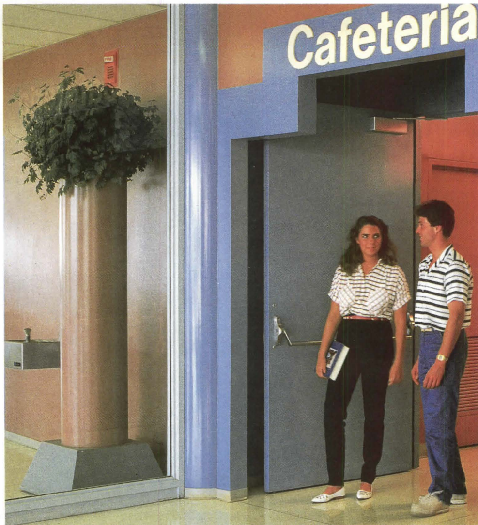
Smoke-activated door closers installed at the College of DuPage Student Resource Center, Glen Ellyn, Ill., prevent the spread of fire by closing doors when smoke is detected.
