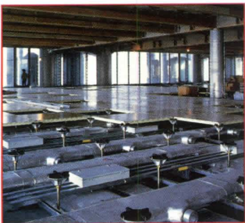
11 Installation of raised floor/HVAC
