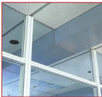
15 Head detail of an interior partition
