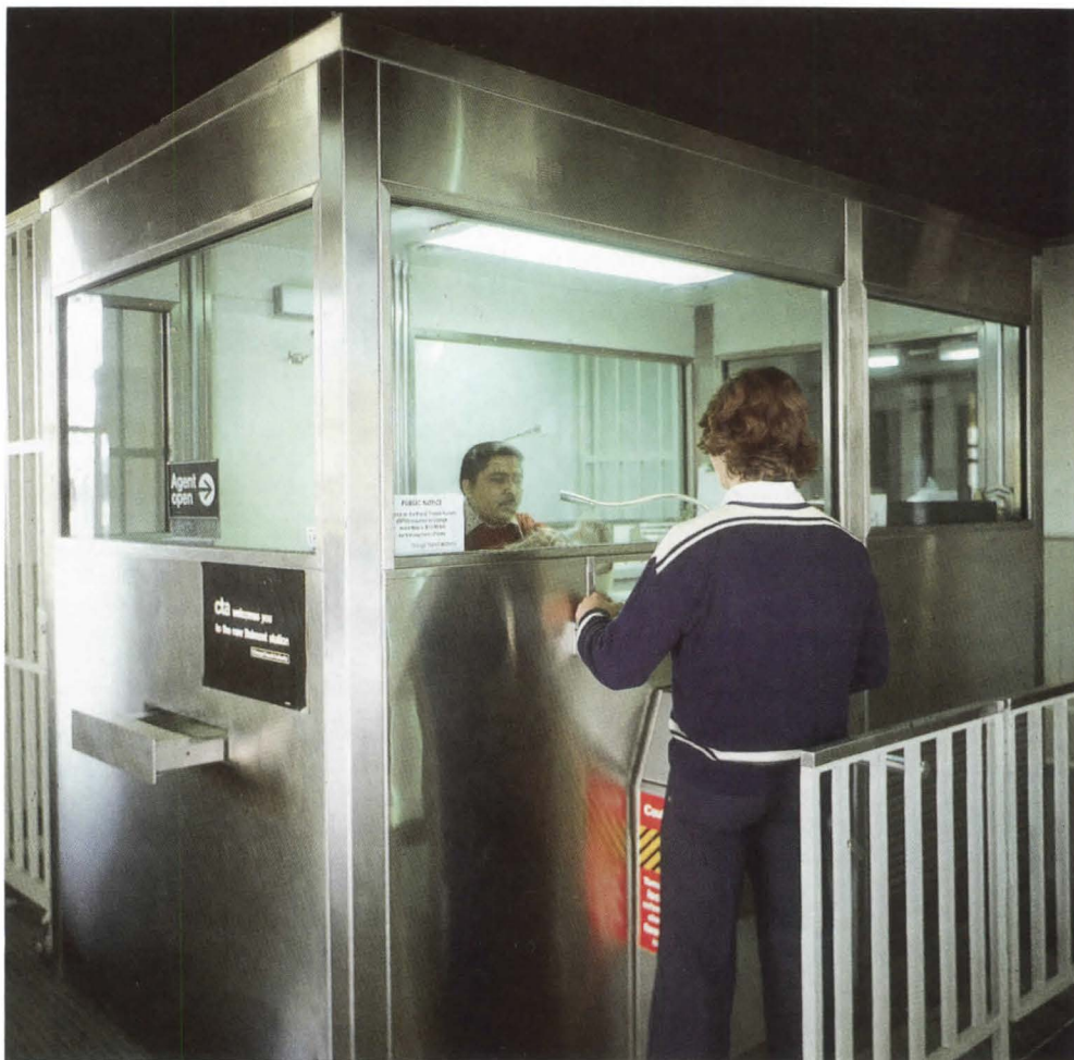
Bullet-resistant materials such as those in this transit station ticket booth were used to provide security at the new sales booth at Metro Center Station, Washington, D.C.
