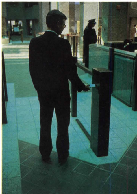
Proximity card readers at One Bell Center, St. Louis, scan employee passes with a beam of light.
