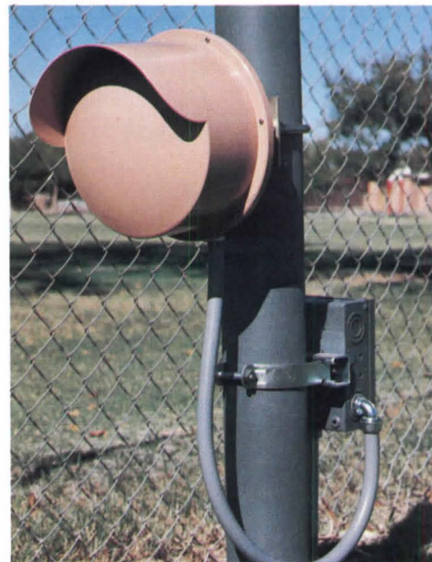
Microwave transmitters like the one above provide perimeter security at Montgomery Ward Corporate Center in Chicago.
