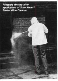
To restore the original appearance of your masonry building, turn to Sure Klean®. Offering over 20 specially formulated restoration products for cleaning tile, terrazzo, brick, marble, stone, terra cotta and most other masonry surfaces. Requiring only a simple cold water rinse, Sure Klean® Restoration Cleaners are easy to apply. Safer to the surface, more efficient and cost-effective than sandblasting or steam cleaning.
