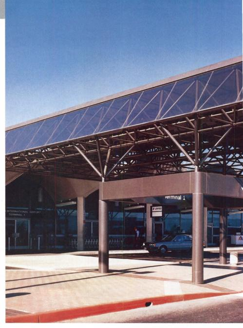
Unistrut System III. Simple node/tube assembly. Allows extra-ordinary design flexibility and latitude, and long-span capability.
