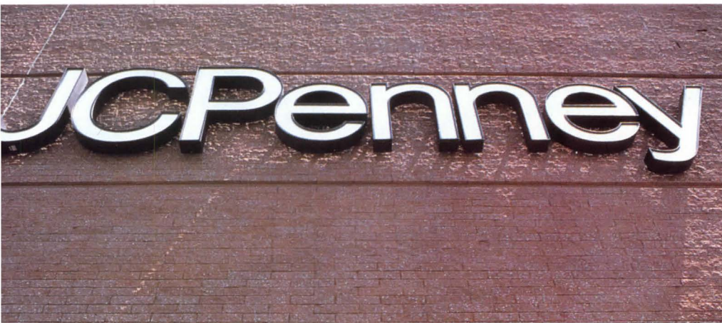
Facade of the J.C. Penney store, one of four department stores in the Mall, is designed in split face concrete masonry units.
