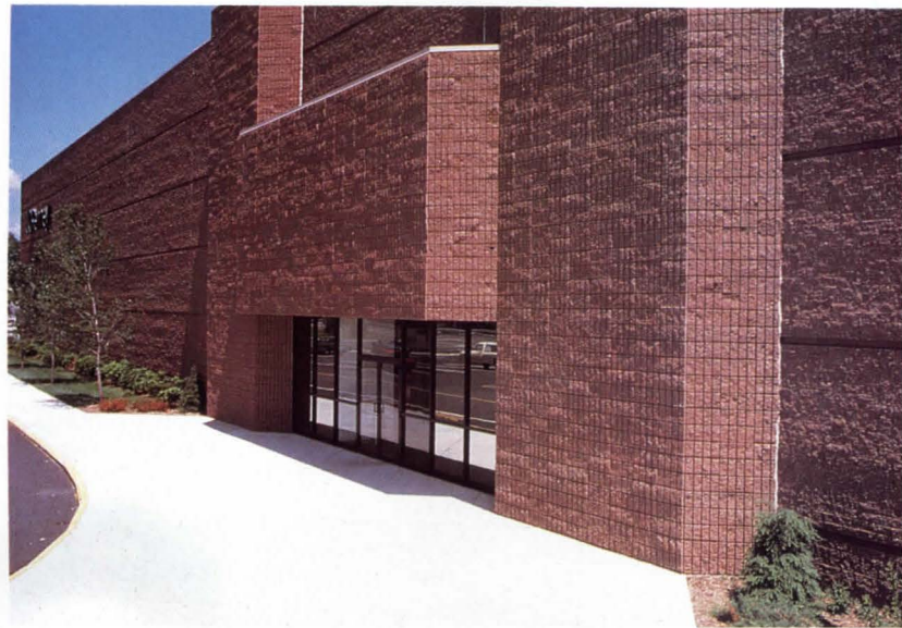
Split ribbed integrally colored concrete masonry delivers a handsome counterpoint to the split face units.
