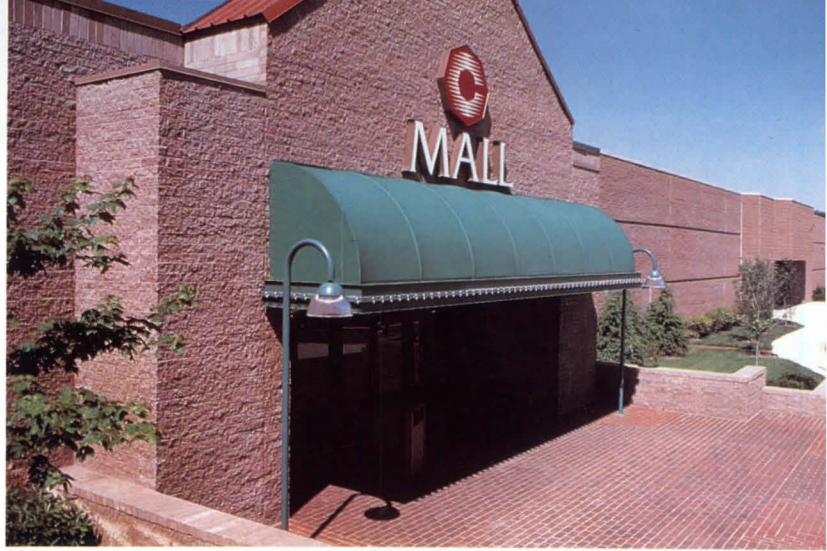
Mall entrance designed in integrally colored split face concrete masonry.
