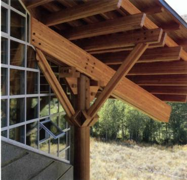
on craft and alpine tradition. **Structural system:** concrete foundations and lower walls; glued laminated beams, purlins, and decking on redwood columns.
