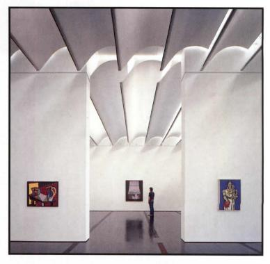
A view of the Contemporary galleries (facing page) shows the building's 20' x 40' bays unobstructed. Similar bays in the Modern galleries (above) are subdivided by removable partitions. Overhead, the "leaf" canopy permits views of north sky through the glazing above (section below); lower edges of leaves have continuous lighting tracks. Stained pine floors include
