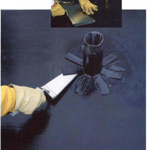
Seaming trowel (above) and flashing plate (top).
