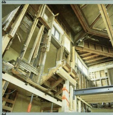
mezzanine floor," says Vinci, "is now about 12 inches rather than 4 inches thick and supported completely by steel. The chains are now fake."
