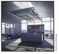
metal ceilings, parts of which have been adapted to serve as radiant heating conductors at the perimeter. The baffles over the podiums are designed to minimize direct glare and to provide indirect light at all times. Jahn and Nada Andric, Murphy/Jahn's interior design director, wanted to avoid the cliché of using United's orange, red, and blue logo and plane trim colors; the leaders at United agreed, and the colors do not appear in the facilities.
