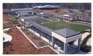
Galvalume sheet offered the Center's architects a way to precisely and cost-efficiently match the color of the arcade roof to the building's charcoal gray trim, enhancing the visual unity of the Center's landscaped approach, arcades and main building.
