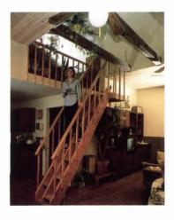
The Wood Lapeyre Stair is crafted in furniture-quality fir with oak treads. It is suitable for difficult-to-reach areas. Each alternating tread provides users with a 10-inch-deep step for secure footing. There also are steel and aluminum models. Lapeyre Stair, Inc.
