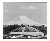
Wood domes like this company's Tacoma Dome offer advantages such as ground-level assembly, construction savings of up to 20 percent, and large clear spans for interior flexibility. Diameters can range from 80 to 800 feet. Western Wood Structures, Inc. Circle 234 on reader service card
