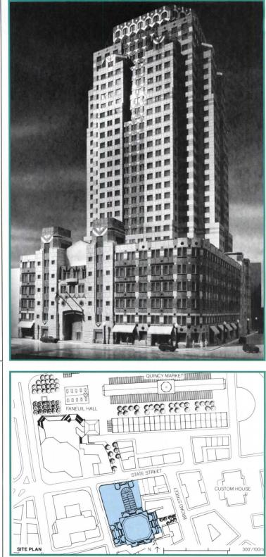
75 State Street, Boston. Architects: Graham Gund Associates, Cambridge, and Skidmore, Owings & Merrill, Chicago. This 715,000square-foot mixed-use complex will be clad in five different types of granite-with polished or flame finishes-supported on steel trusses. The 31-story, setback office tower rests atop 40,000 square feet of street-level retail space rendered in red and gray-beige granite. The main entrance leads to a six-story courtyard atrium and grand hall clad in five different marbles,
