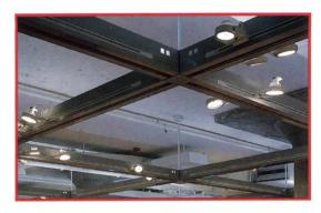
The showroom's lighting system (detail, left) is a network of six-inch-square-section channels on a ten-foot grid. **Each channel contains** fluorescent uplighting to illuminate the ceiling, while incandescent track lights fit into the sides of the channel; the two types of lighting are individually adjustable. The small squares cut into each channel indicate when the
