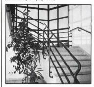
Custom railing, for indoor and outdoor commercial and residential installations, is made of tubular, nylon-coated steel that is warm to the touch, easy to maintain, and strong. The railings are suitable for handrails, safety rails, or curtain rods in schools, hospitals, offices, and residences. They are available in 12 colors and coordinate with other company products including shelves, handles, grab bars, and locking systems. Normbau, Inc.
