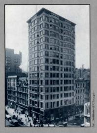
Chicago's Reliance Building, an important early high-rise designed by Burnham & Root, is threatened less by outside forces than by the poor condition of its terra cotta façade, which is cracking and is tenuously attached to the building frame. The city government has pledged \$2 million to help finance restoration. Still, the costs involved in restoring the two great terra cotta walls may be more than the building's rental income potential will justify.
