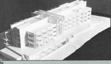
The skin of this building is made of silver-colored metal panels with painted tube steel and curved stainless steel screens. A grid of vertical granite planes divides the building into quadrants; a superimposed diagonal system directs circulation. Between the stone slabs are skylighted atriums.
