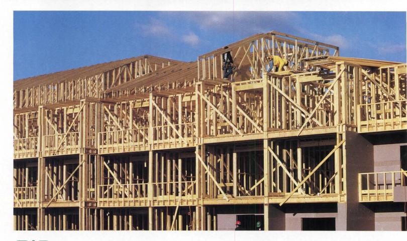
hen Marriott Corporation switched to engineered wood systems for their Courtyard Hotel near Washington, D.C., they saved about \$100,000 in materials and labor costs—about 10% compared to the firm's previous masonry and steel design.
