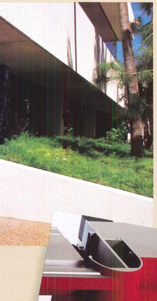
Radiused borizontal and vertical framing members present a softly sculpted interior. Crystaline is a smooth, continuous exterior of uninterrupted reflective glass. With no visible mullions or metal framing.
