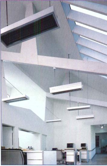
At the point where one of the gables turns into a simpler shed roof, the two canted clerestory windows (left, top two photos) occur in the Housing Support Services open office area; they are emphasized because this is the function that Moss sees as the most important of the office uses. Ductwork in the building (left, bottom) was given special attention, resulting in
