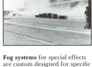
applications. They utilize direct pressure nozzles to generate microscopic water droplets so small that they float in the air. The system is offered preassembled with pumping and filtration components. Mee.
