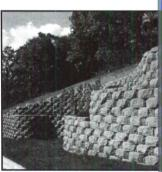
Retaining walls may be specif in three sizes, with different fa patterns and angles, and in a variety of colors. Standard unit weigh about 94 pounds. Keystone.
