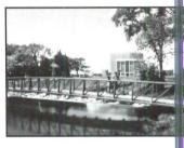
Pedestrian bridges are constructed of tubular, weathering steel, painted carbon steel, or highly corrosion-resistant alu num. Custom designs can be fabricated for a variety of use Continental Custom Bridge. Circle 116 on reader service card
