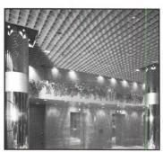
A new ceiling system called Cube Ceiling features a oneinch-deep cube. Crossbeams are inserted at right angles to the suspended hanger sections and factory assembled lay-in cubes are fitted into the resulting grid. An acoustical mineral board lid is an option. CDA.
