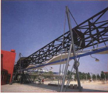
VIEW OF BOX FRAME SHOWING CABLE SUPPORT AND STIFFENER
