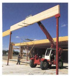
The cost efficiency of panelized wood roof systems means less construction time. These glued laminated girders span from 27 to 30 feet.
