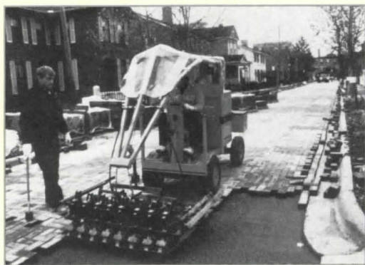
MECHANIZED INSTALLATION WITH CUTTING OF EDGE UNITS.
