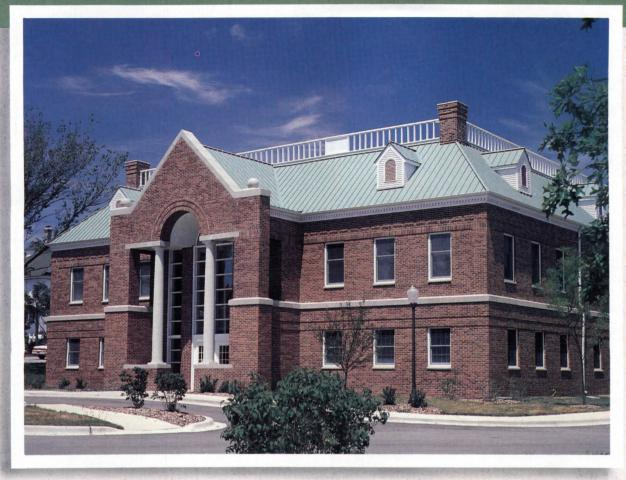
Integral Standing Seam .032 aluminum 24 gauge steel 11", 18" or 19" O.C. 11/2" high
