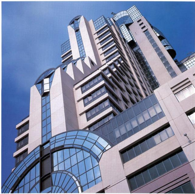
Precast concrete construction with Lehigh White Cement offers the architect unlimited freedom for creating sophisticated contemporary designs with functional advantages and construction economies.
