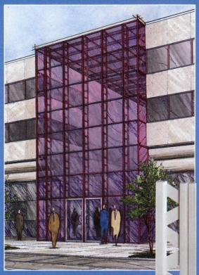
But while the design options offer flexibility, the integrity of the structure remains inflexible. A thermal break, and the flexibility of either  $\frac{1}{4}$ " or 1" glass attest to Trusswall being ready and willing to take on nature's harshest elements.
