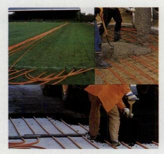
Installs quickly and easily under concrete and asphalt, or in existing turf.
