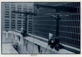
Workers position davit into roofmounted socket (left). Davits may also be mounted on rails secured to parapets (right). This self-propelled roof car (right) has integral counterweights and can be clamped to its track to resist overturning.
