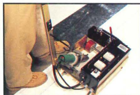
Self-propelled, hot-air welding machine fuses HyChoice seam.
