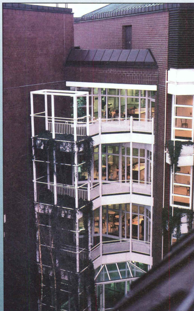
The Colonia Insurance Headquarters by BHLM in Germany demonstrates a renewed focus on landscaped views for every workstation, natural ventilation, and operable shading devices.
