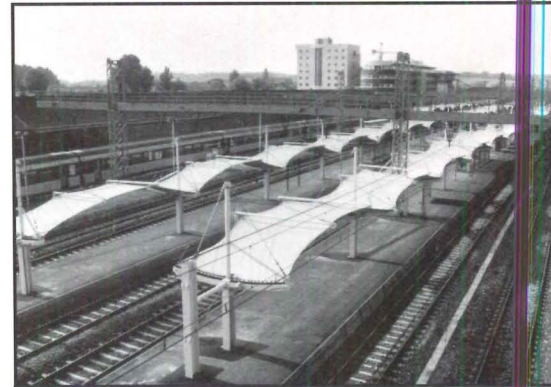
Platform shelters at TGV's Le Mans station.
