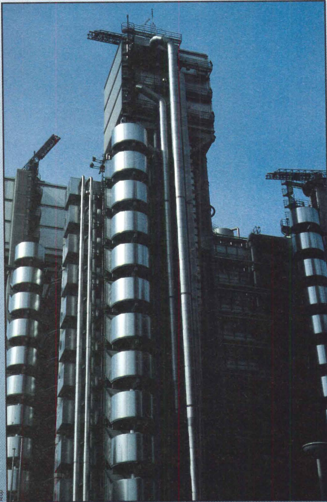
Lloyd's of London by the Richard Rogers Partnership reveals dedication to technical system aesthetics and dynamics with exposed exterior cores and air-flow windows.
