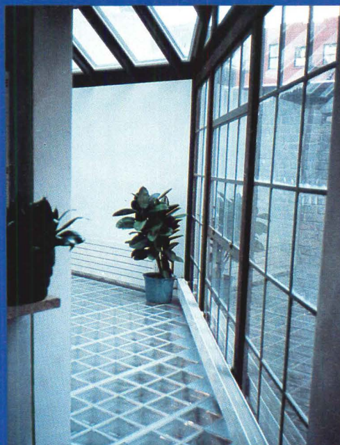
Residence Dining Room Floor Solarwhite Glass Block & Aluminum Assembly New York City Architect: ACBC Associates, New York
