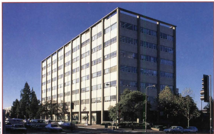
University Hall's nonductile columns needed bracing for better seismic performance (northeast corner view).
