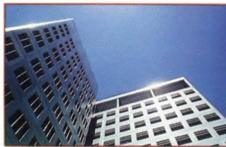
The building as a natural heat exchanger: Champion International Headquarters, Stamford, Connecticut, by Ulrich Franzen, architect. Each side of the building has a different sun-shading system, optimized for its orientation. Horizontal louvers on the south admit winter sun and reflect daylight on interior ceilings.
