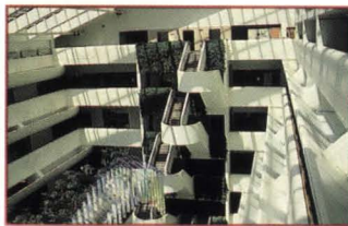
The building as a natural light diffuser: TVA Headquarters Building, Chattanooga, Tennessee, by the Architects Collaborative. The cross-section and interior atrium are designed to maximize natural lighting.
