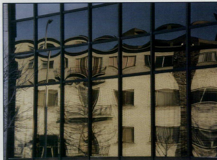
1, 2 Visual distortions are caused by changes in temperature and barometric pressure, which cause glass lights to bow in or out.
