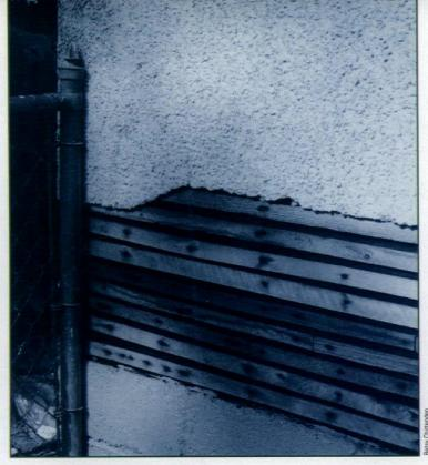
EMOVAL OF DAMAGED STUCCO PRIOR TO REPAIR
