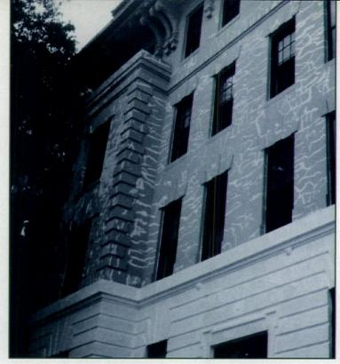
THE EFFECT OF CAULKING STUCCO CRACKS
