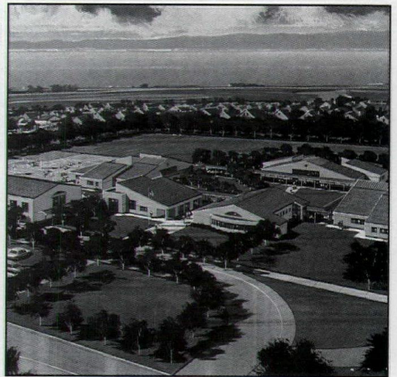
VIEW FROM NORTH
