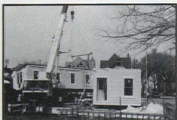
Modules are set on the foundation with a crane in one day.
