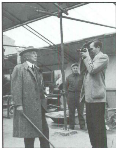
On site at the Guggenheim Pavilion, 1953.
