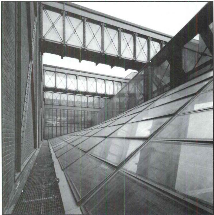
WARP IN SKYLIGHT AND RESULTING GLAZING PLACEMENT
