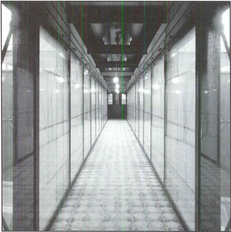
BRIDGE, FRITTED WALLS, AND GLASS BLOCK FLOOR
