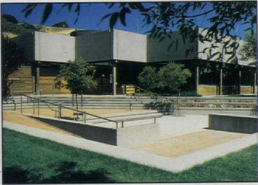
View From Southwest
