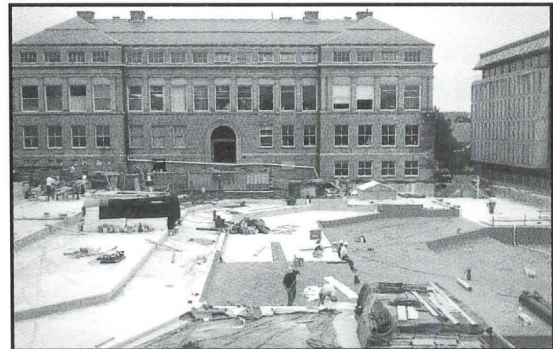
1 The Carl L. Kroch Library, a new addition to Cornell University's central library designed by Shepley Bulfinch Richardson & Abbott, is buried beneath the lawn in front of the older building. 2 During construction at the library, the underground addition's stepped-roof profile can be seen.
