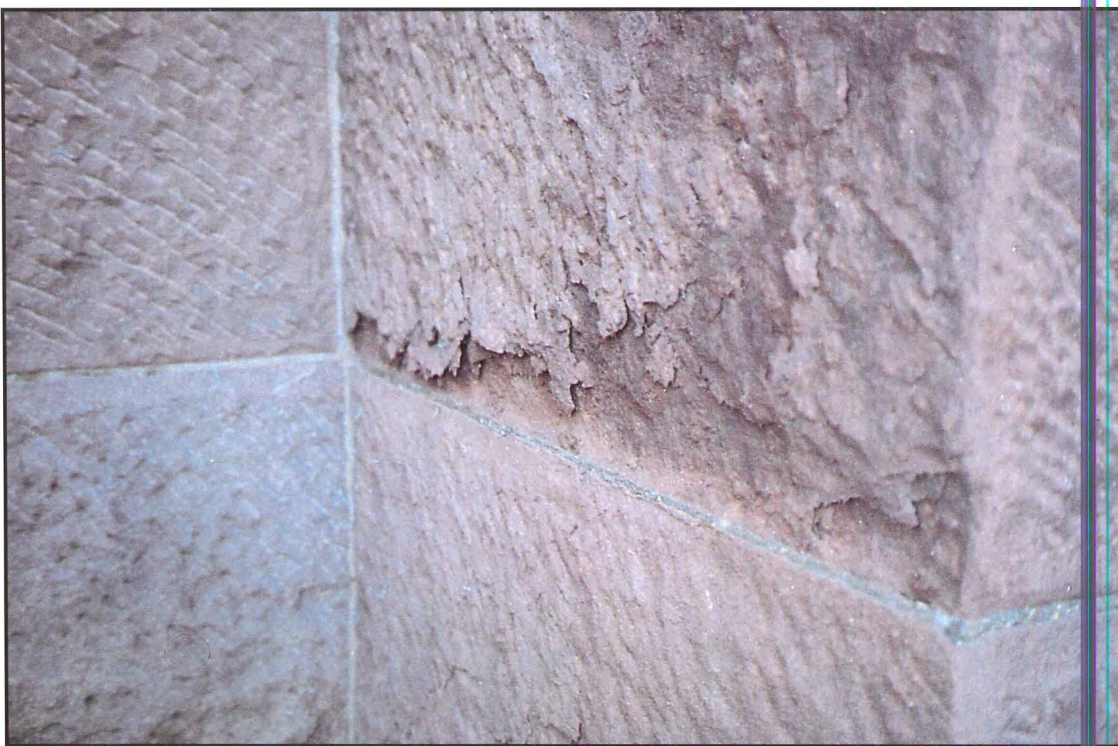
2 SANDSTONE SPALLING BECAUSE OF POOR BEDDING PLACEMENT
