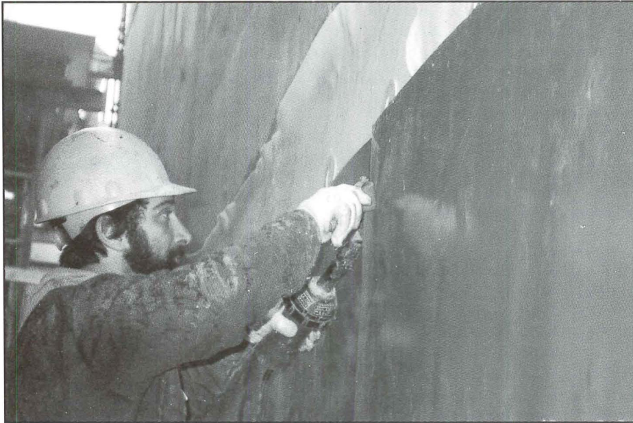
7 HEAT-WELDING WATERPROOFING MEMBRANE TO ATTACHMENT DISKS
