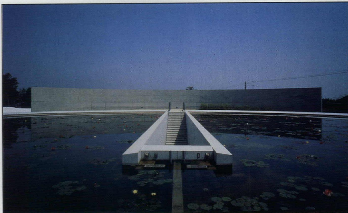
1 CURVED CAST-IN-PLACE CONCRETE AT ANDO'S LOTUS TEMPLE
