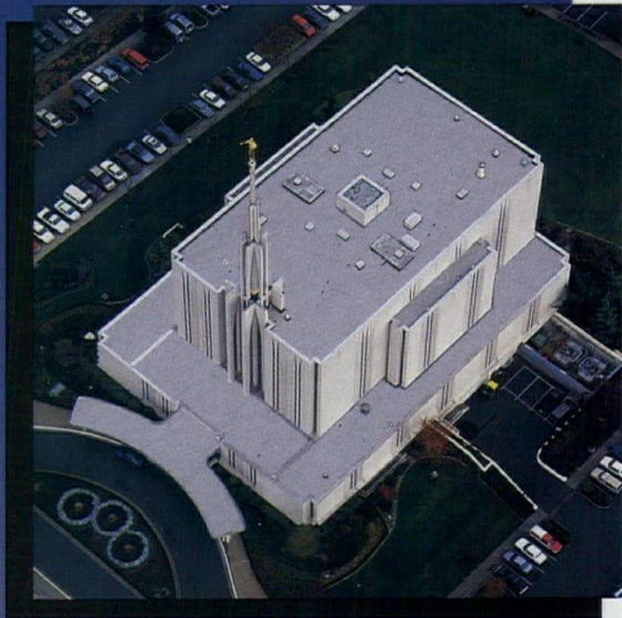
Above: LDS Temple, Bellevue, WA Carlisle SynTec EPDM roofing system Roofer: All Weather Waterproofing
