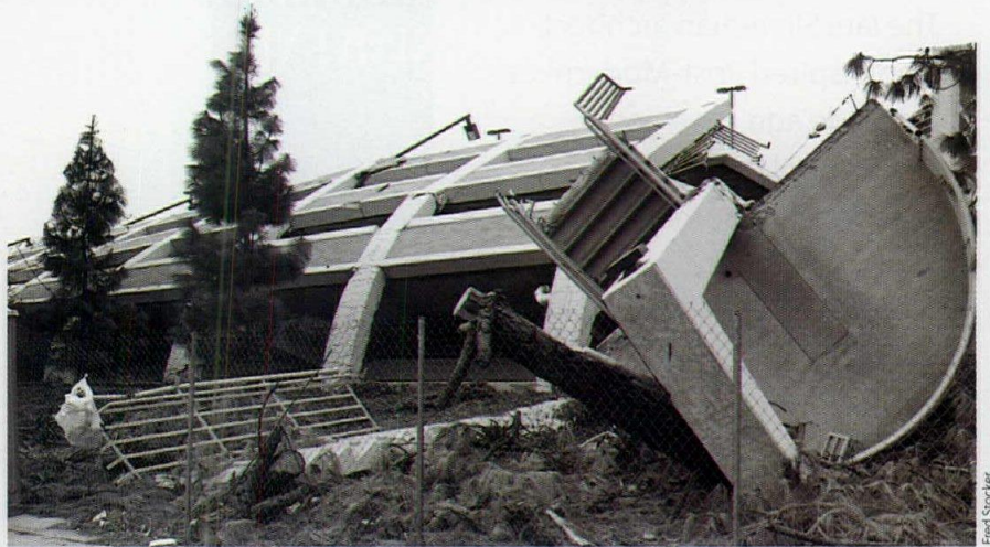
Of all recently built structures, parking structures, like this one at California State University at Northridge, were the most vulnerable, because of the extraordinary loads that roof decks exerted on widely spaced columns. Most of the collapsed parking structures lacked shear walls.
