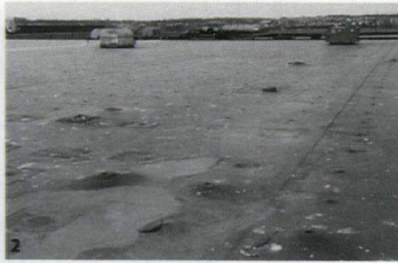
2 Suction at the base of a wall can cause screw fasteners to pull free or back out.
