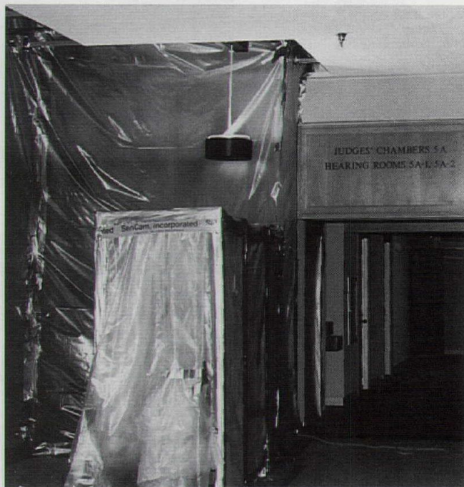
4 POLYETHYLENE BARRIERS ISOLATE MOLD SPORES FOR REMOVAL
