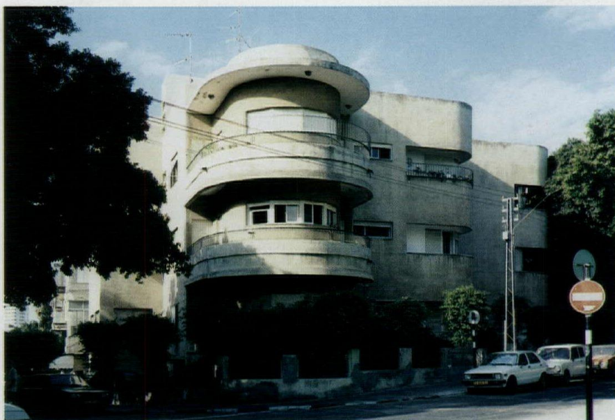
A typical four-story apartment building, designed by architect Pinhas Hüt, displays Mendelsohn's influence.
