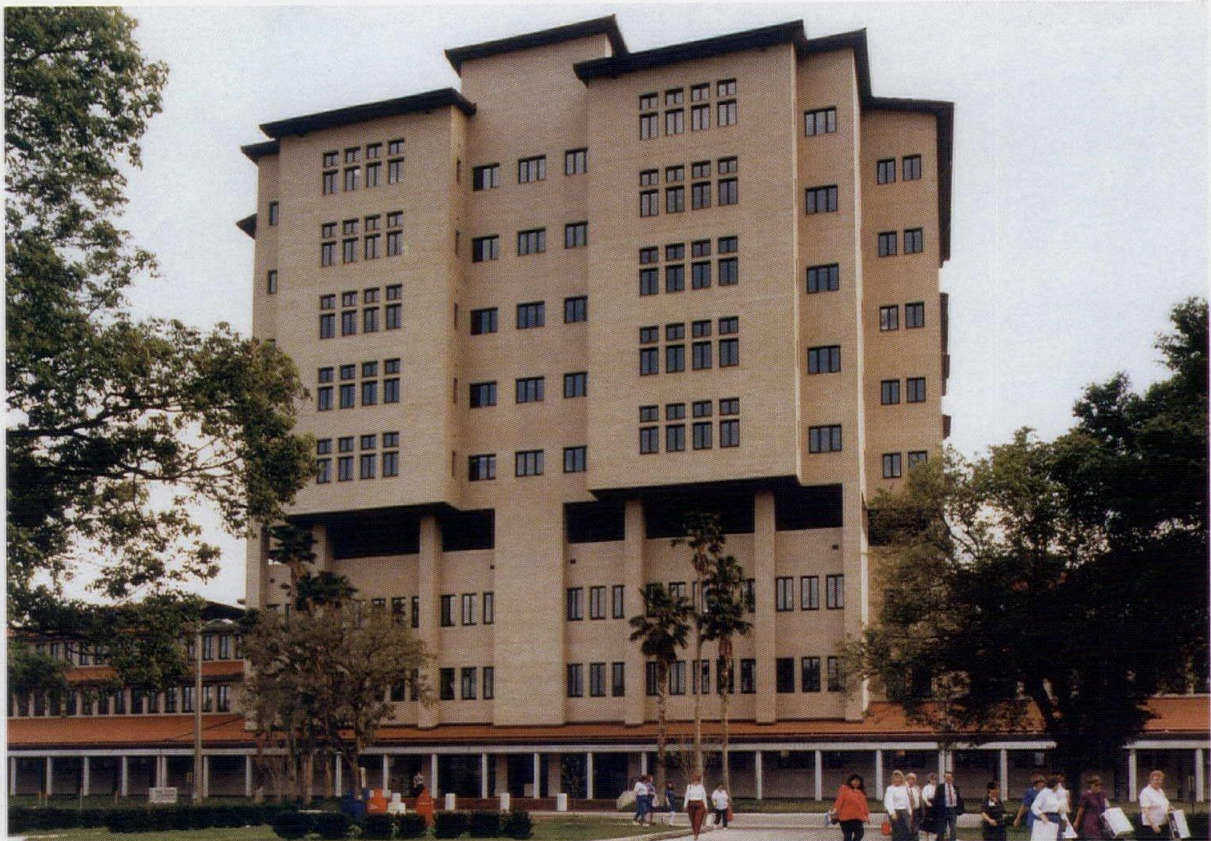
2 IMPERIAL POLK COUNTY COURTHOUSE EXTERIOR
