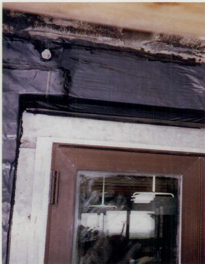
3 RUBBERIZED ASPHALT MEMBRANE INSTALLED AROUND WINDOWS
