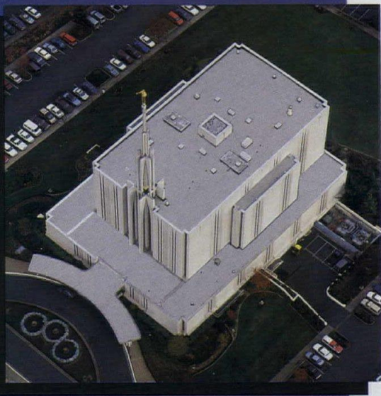
Above: LDS Temple, Bellevue, WA Carlisle SynTec EPDM roofing system Roofer: All Weather Waterproofing
