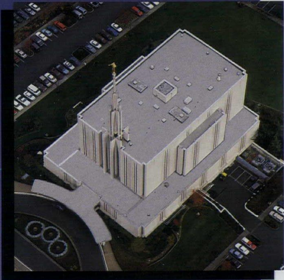
Above: LDS Temple, Bellevue, WA Carlisle SynTec EPDM roofing system Roofer: All Weather Waterproofing
