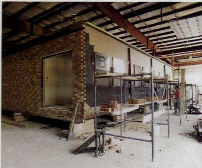
VIEW OF TYPICAL FACTORY ASSEMBLY AT KULLMAN INDUSTRIES
