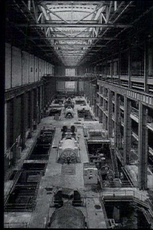
EXISTING TURBINE HALL
