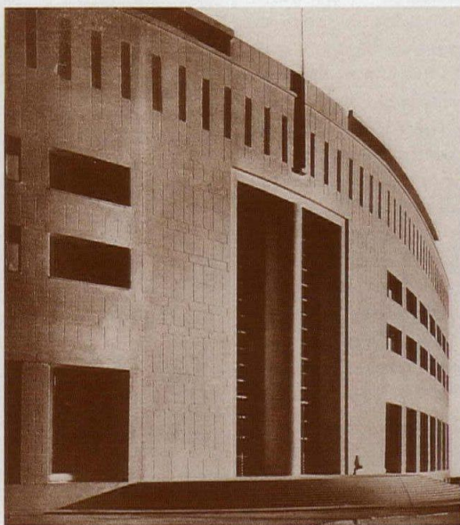
Naples Post Office, designed by Giuseppe Vaccaro. Mussolini reportedly liked the design; "the curious split entrance," wrote Nelson, "is a typical example of the persistent use of the fascist symbol." But "the Neapolitans saw nothing but indecent nudity" in the scheme.
