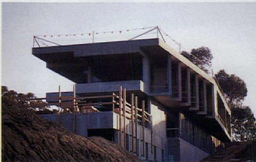
THEORY CENTER UNDER CONSTRUCTION VIEWED FROM NORTHEAST
