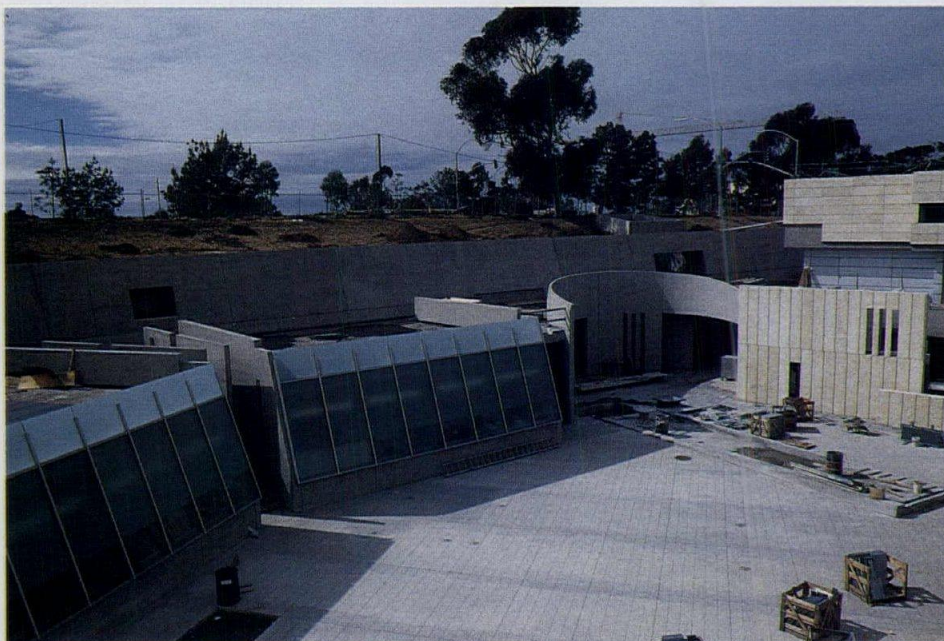
COURTYARD AT JUNCTURE OF LABS AND THEORY CENTER
