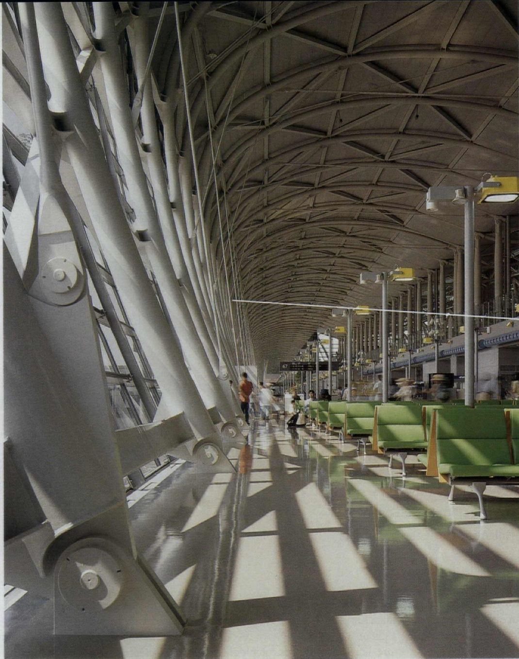
Along the field side of the terminal, the swooping roof wraps around to meet the floor at the second level, generating a tubular boarding lounge volume that extends, with diminishing height, to the extremities of the boarding wings. An impressive display of crisscrossing steel members is accentuated by daylight from the field.
